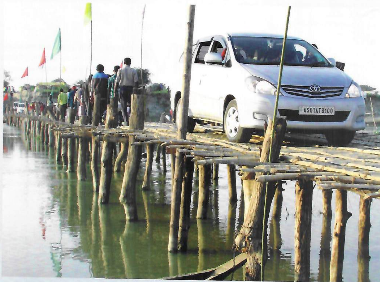
Construction of Cold Weather Bridge at Disangmukh
