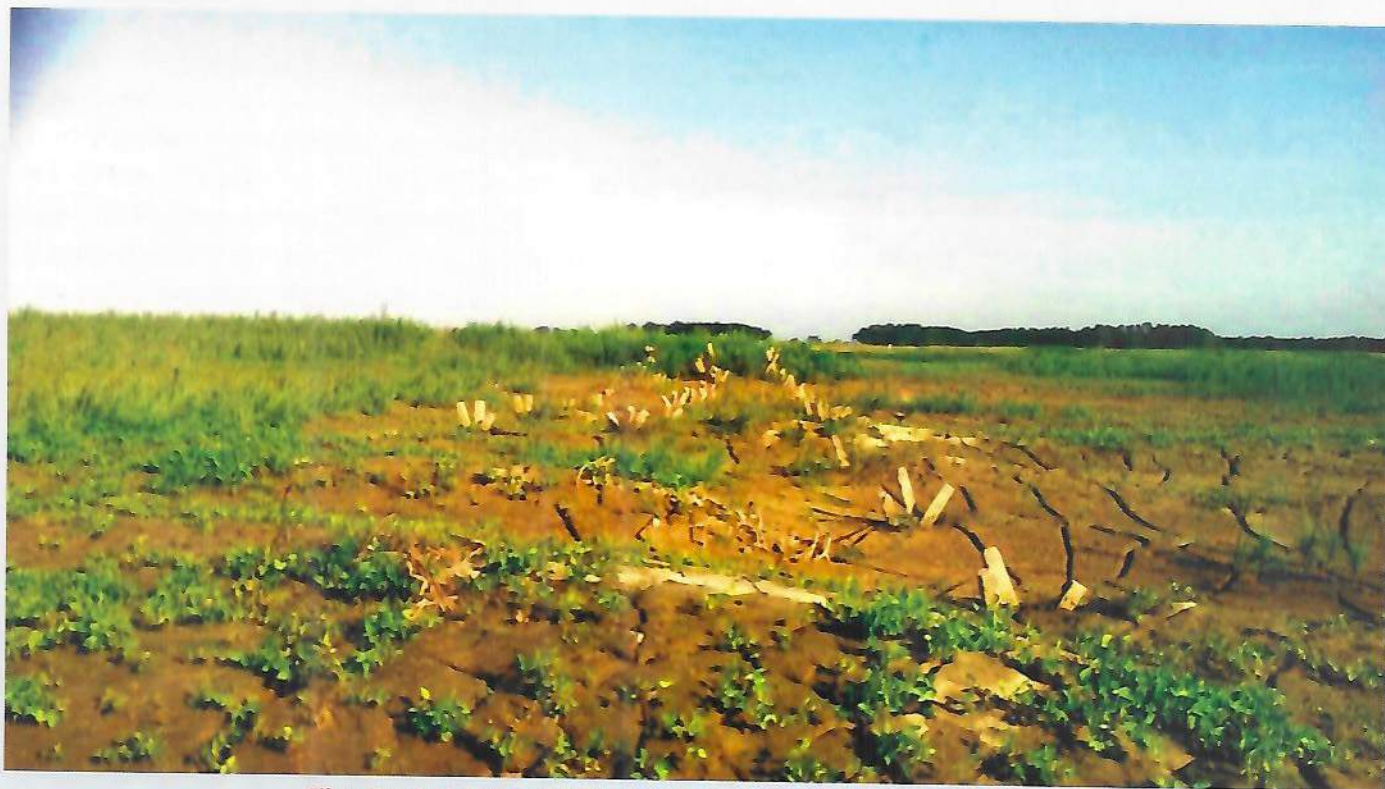
Siltation induced by RCC Porcupine Screen at Dhansrimukh, Bokakhat
