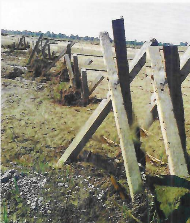
Successful Siltation Induced by RCC Porcupine
