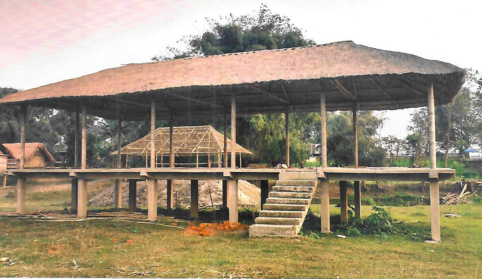
A Murong with RCC Posts and Beams
