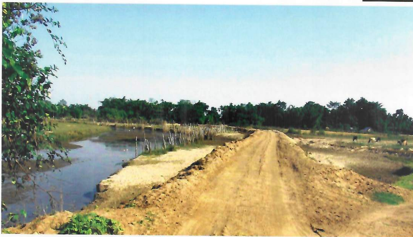
Construction of Guide Bundh from Majorbari to Burisuti River
