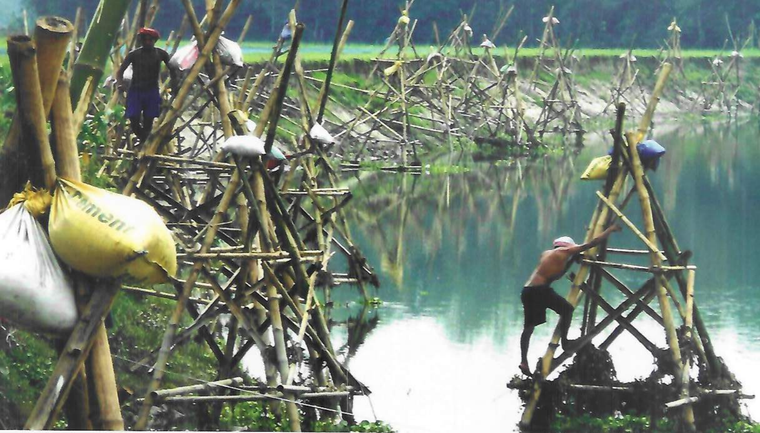
Erosion Protection Work with Bamboo Cribs at Kolani on Kherkota River (Luhit Pashim Constituency)
