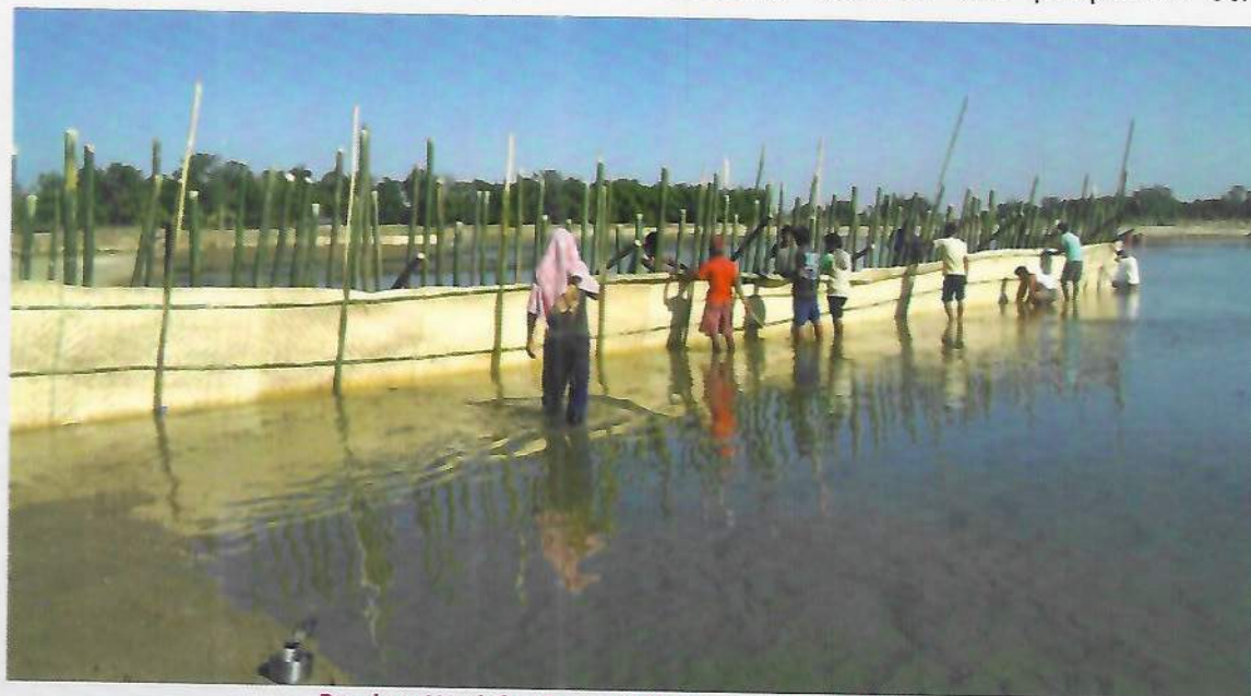
Bamboo Work for Current Diversion of Jiadhal River
