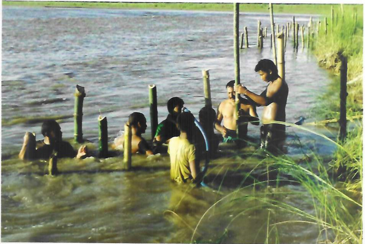
Bamboo Work to Control Jadhah River at Dihiri Village
