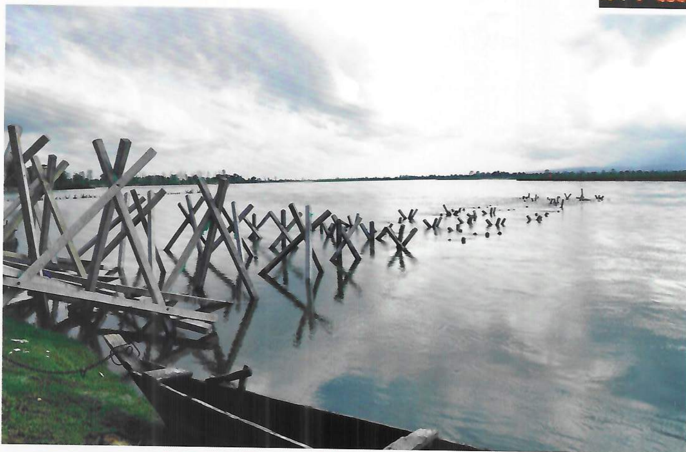
RCC Porcupine Screening on Subansiri River for Erosion Protection
