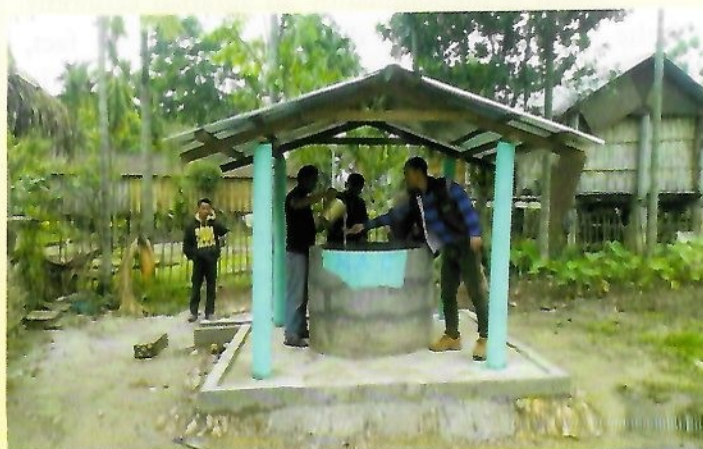
Installation of Ring Well complete with CC floor, Drain & Soak Pit in MAC areas
