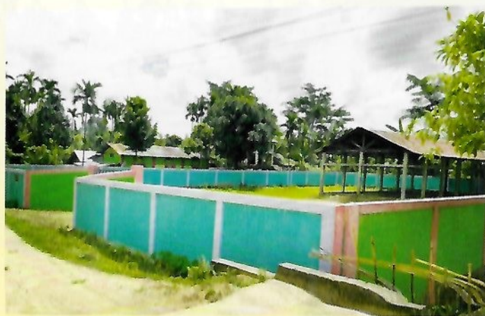
Construction of boundary wall and land development of Mohonpur Tulungsi Club campus (Sanjari Nwngwr)
