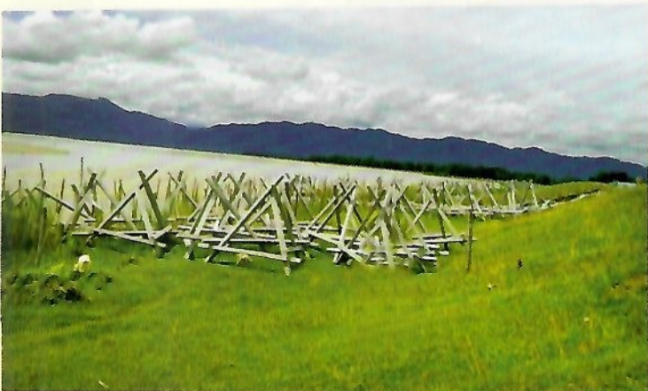
Erosion protection with RCC Porcupine screening
