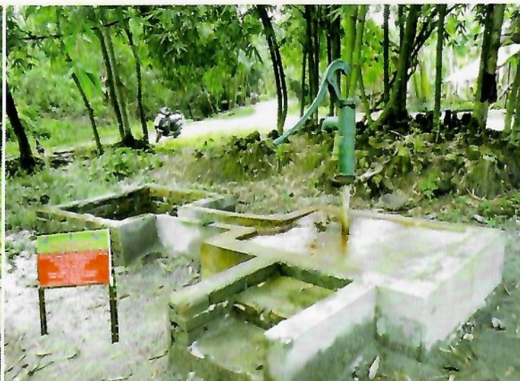
Installation of Hand Tube Well complete with CC floor, Drain & Soak Pit in MAC areas
