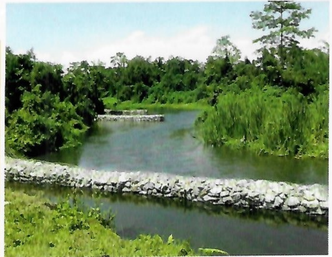
Erosion protection with Boulder Spur
