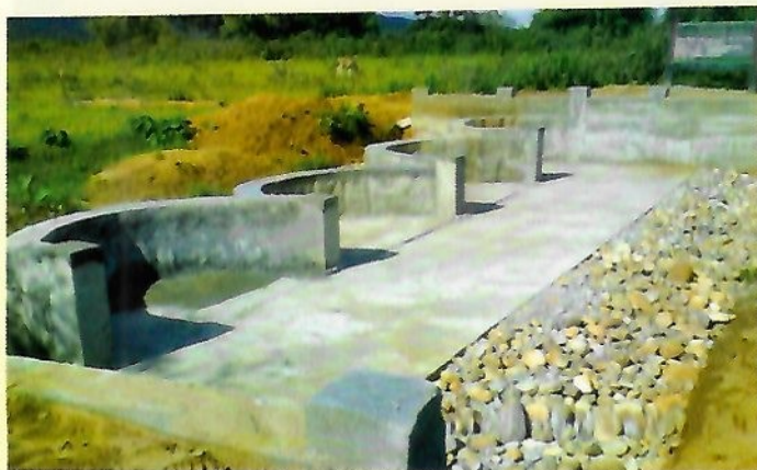
Construction of Gully Control at Chiloni Jan (Nalbari Constituency)
