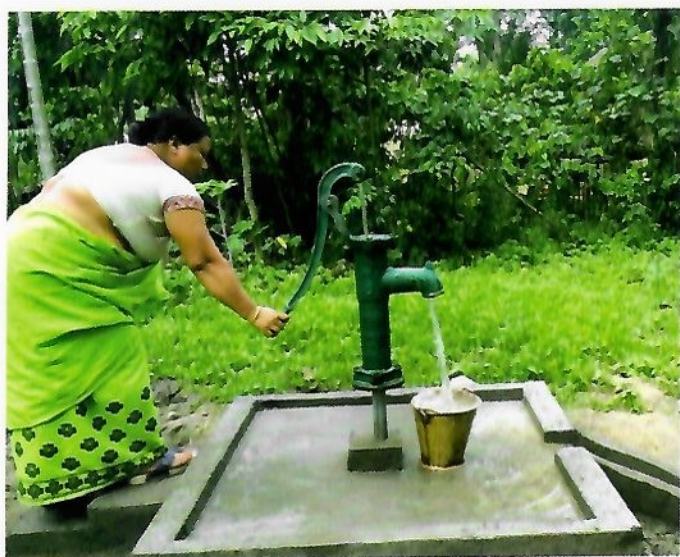
Installation of Hand Tube Well complete with CC floor, Drain & Soak Pit in MAC areas
