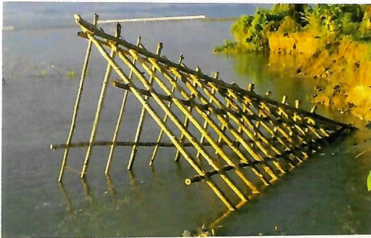
Erosion protection work by Bamboo Triangular Cage
