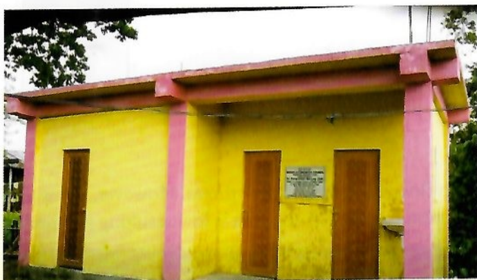
Construction of Public Toilet in MAC areas
